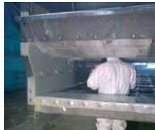
**Lining (Corrosion Protection)**
