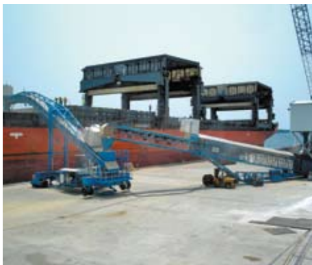
Shiploader – Conveyor Feed
